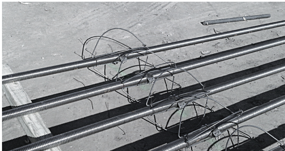
Unispacers attached to all-thread bar
