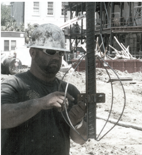
Field installation of Unispacer
