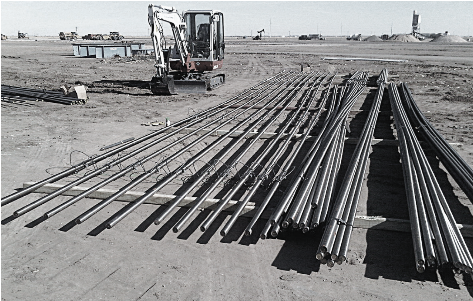
Unispacers attached to staged single bar reinforcement
