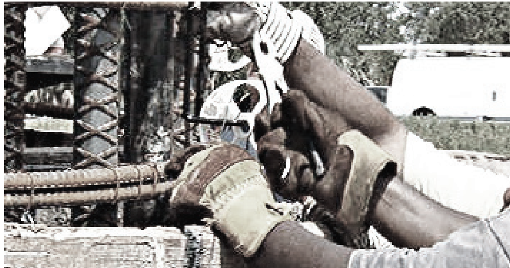
Attaching the Hairpin with tie-wire
