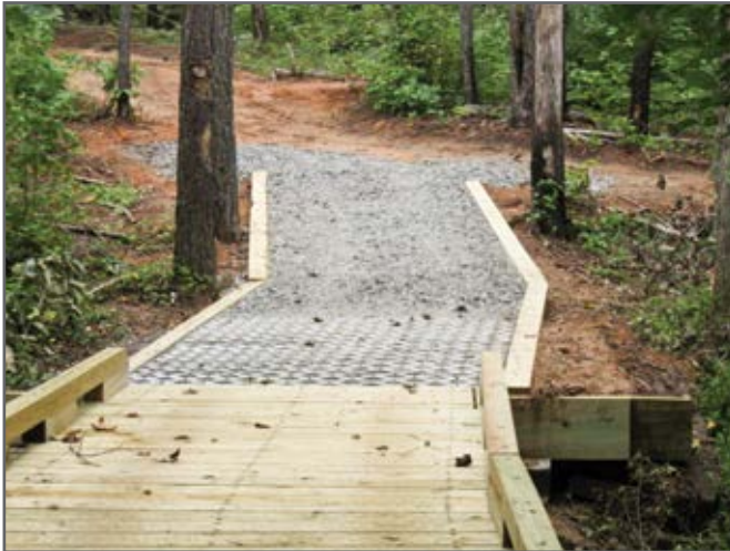
Step 11—Masonry block pavers at the boardwalk approaches provide a firm transition from the trail to the boardwalk and minimize soil settlement.
