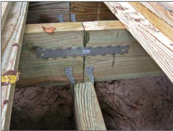
Step 7—Stringers are carefully placed on header beams and Simpson Strong-Tie metal components are used to join members.
