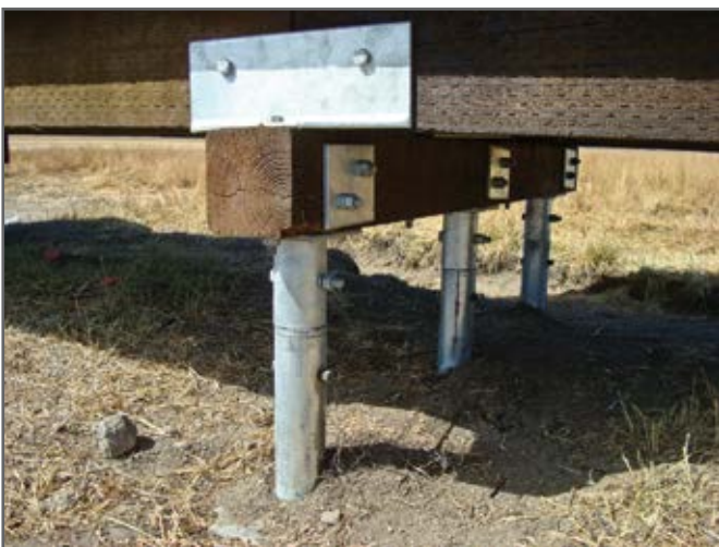
Step 7—Pipe sleeves are used to bolt saddle brackets to the pipes and header beams to form a bent.
