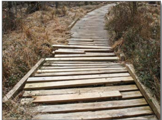
Step 1—The OHV elevated boardwalk is installed during a dry period while accessibility for equipment is good. The first step requires removing the existing deteriorated boardwalk.
