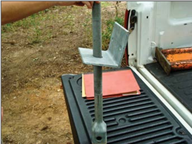
Step 3—Galvanized steel brackets are used for lateral bracing.
