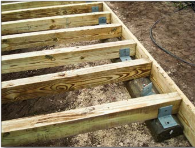
Step 7—The nonelevated end of the structure is secured to a partially embedded plastic curb sill.
