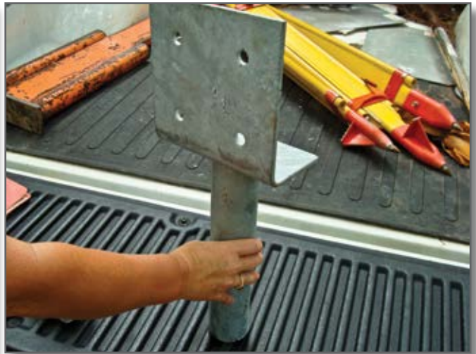
Step 4—Galvanized steel saddle brackets attach to the helical piles and header beams to form a bent.
