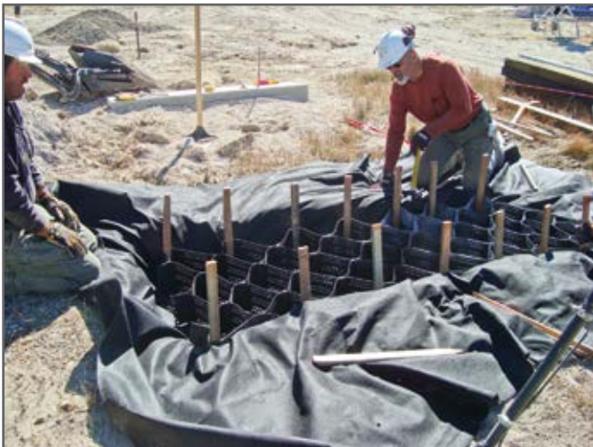
Step 2—Geosynthetic fabric is placed, and the geocell is staked and filled with gravel. Geosynthetic fabric is folded over the top.
