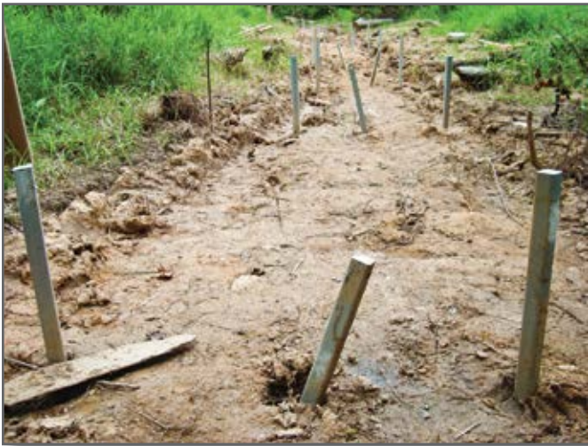
Step 2—Helical piles are installed using a mini-excavator with a special screw head and hydraulics. The contractor installed 90 helical piles at an average depth of 10 feet over 3 long workdays. Helical piles are installed both vertically and at an angle. The direction of the angled piles alternates between bents for lateral bracing purposes.
