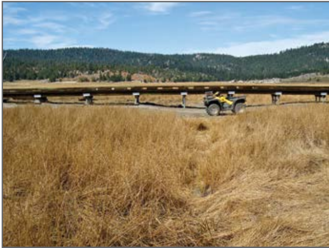
Figure 3—Precast concrete barriers on top of geogrid filled with stone provide solid footing for this Snake Creek Trail boardwalk at the Inyo National Forest in California.
