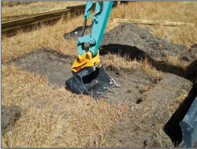
Step 1—A trench 8 feet by 3 feet by 1 to 2 feet (depth depends on the required substructure ground elevation) is excavated to accommodate the wrapped geocell and precast concrete foundation.
