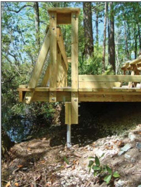
Step 8—The viewing/fishing platform support system.
