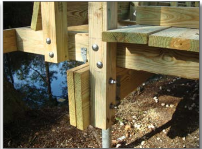
Step 5—The structure is cantilevered 2 feet over the helical piles to allow water to drain off the boardwalk while avoiding the exterior beams. This also allows better access for fishing.
