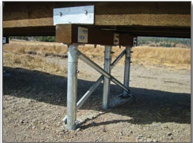
Step 8—Two-inch-wide galvanized steel C-channel cross-bracing is added where the structure is 3 feet or higher above the ground.
