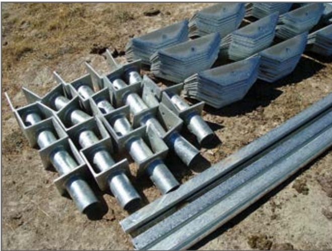
Step 6—Saddle brackets are bolted to the tops of the pipes and 1/8-inch weep holes are drilled at the bottoms to prevent water from collecting, freezing, and breaking the pipes.
