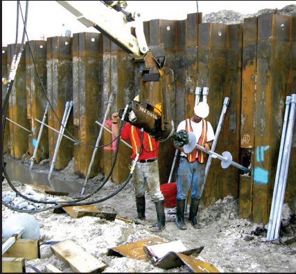
Sheet Piling Shoring
