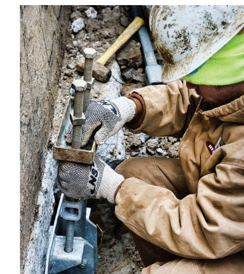
UNDERPINNING INSTALLATION
