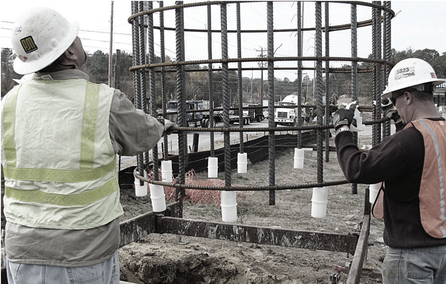
Guiding rebar cage into drilled shaft with Barboots attached
