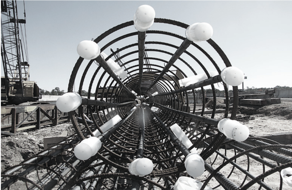
Rebar cage staged with Barboot supports attached
