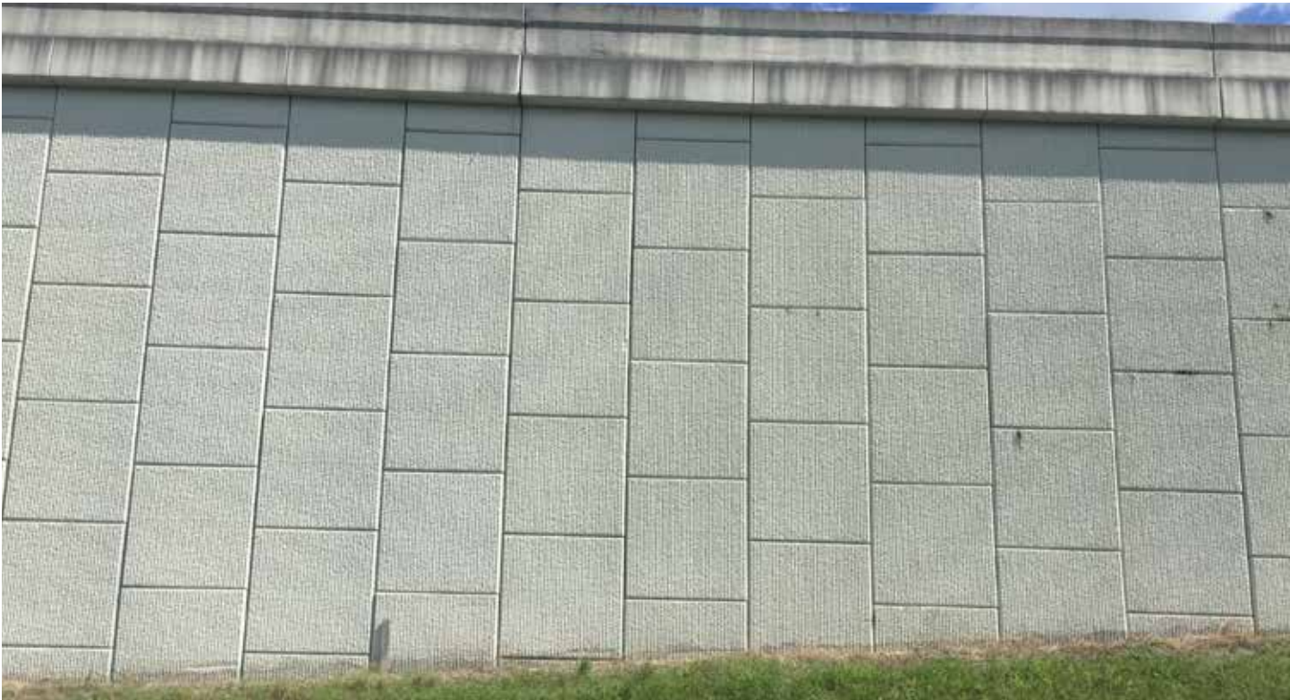
Figure 3: Test Section after the FDS has been installed.
