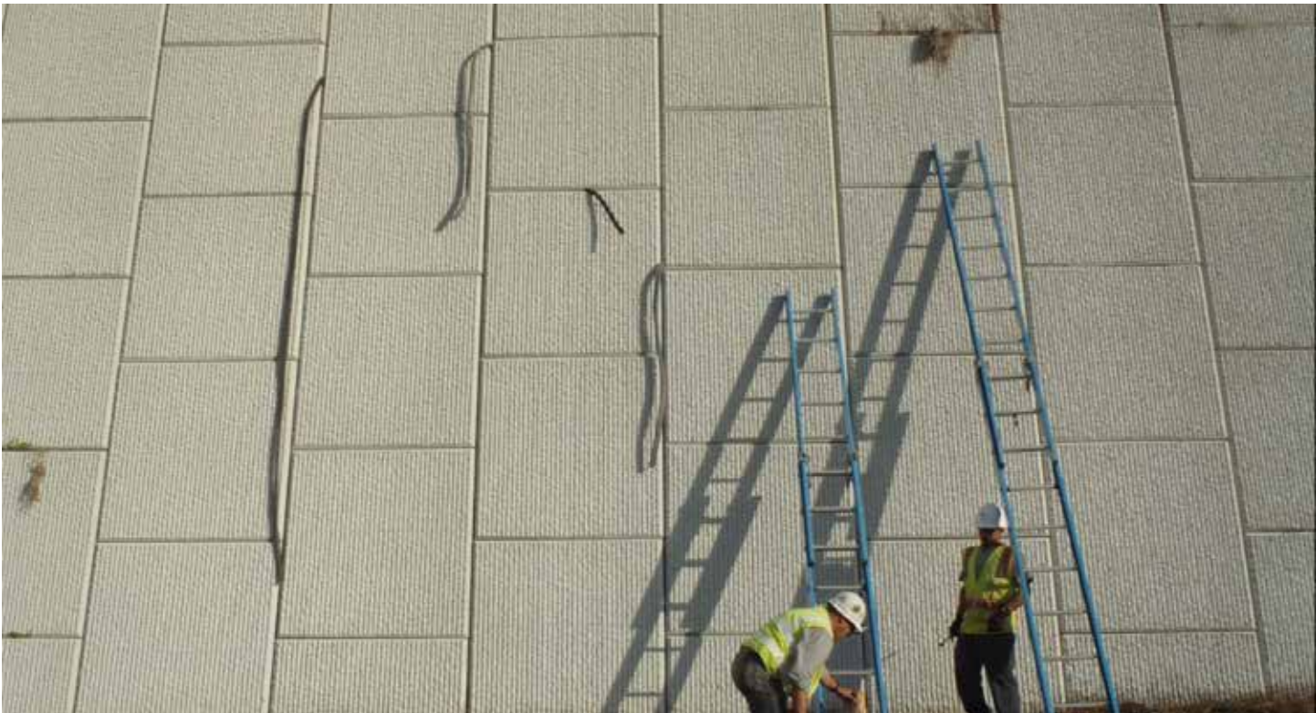
Figure 4: Installation of the FDS product
