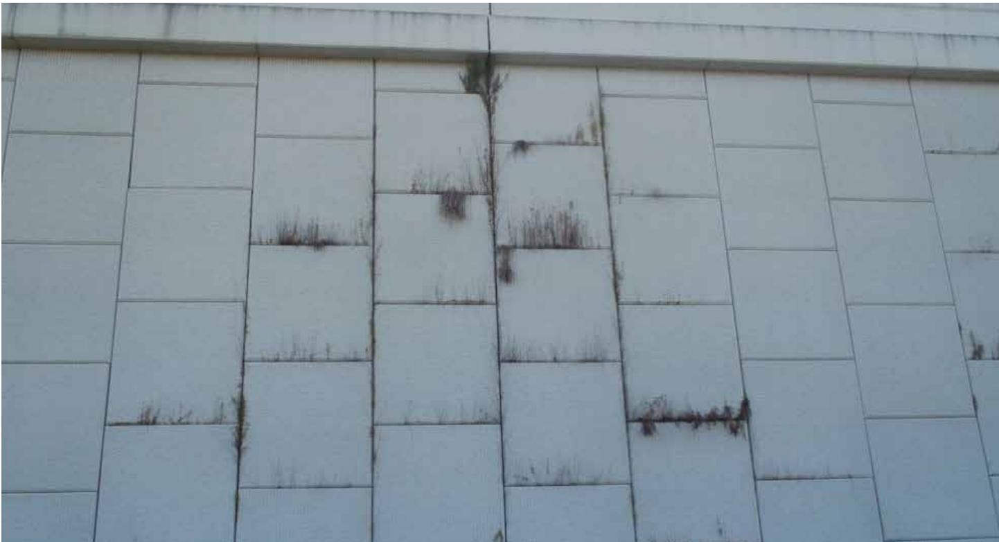
Figure 2: Test Section without FDS prior to vegetation removal.
